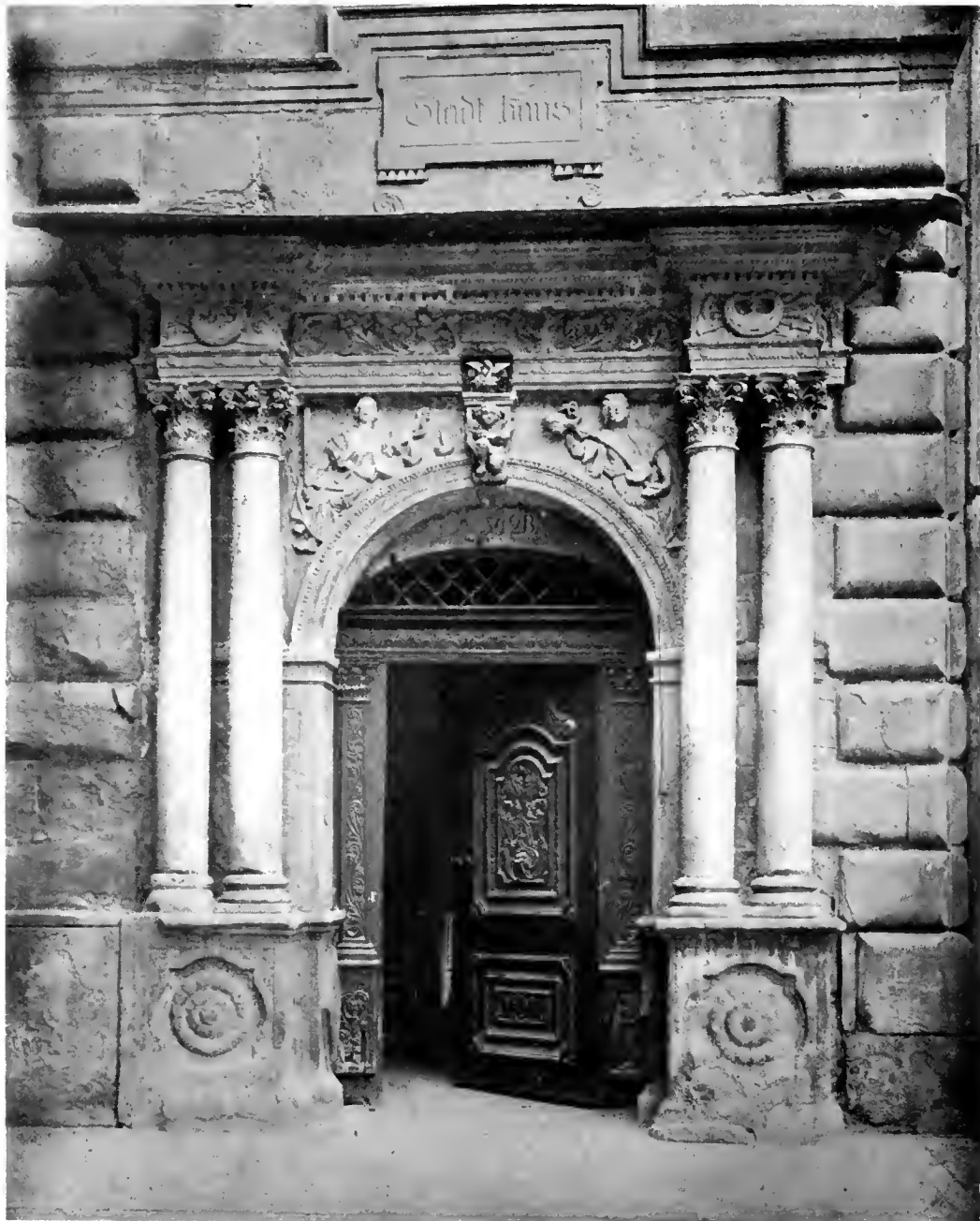
DETAIL OF DOORWAY—RATHAUS, LUCERNE
